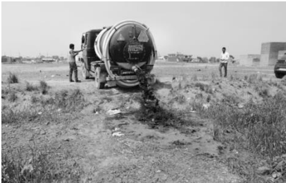
Disposal of untreated wastewater and septage
